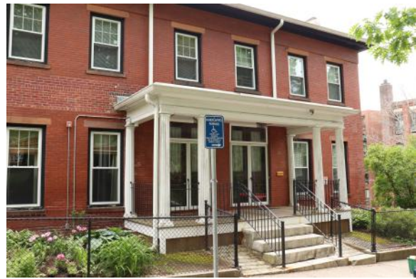
The Abby's House shelter remains largely unaltered since its inception almost 45 years ago.
