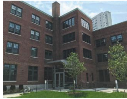
New, accessible entrance into 52 High Street
